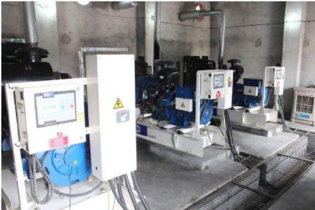
Triple back-up system to ensure an uninterrupted power supply
